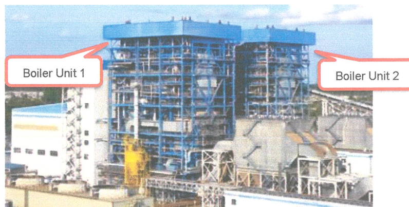
Boiler Unit 1, Elevation 00.0 m (Sampling for References)
